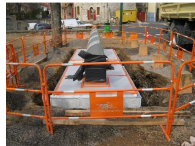
Installation de conteneurs type ECOBIG - St Amand Tallende
